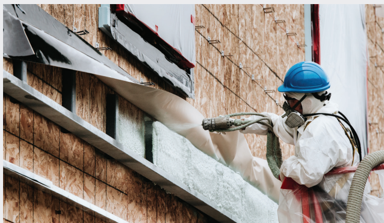
Figure 2: a) PIR board insulation with foil facers (photo courtesy of Pirmax Pty Ltd), b) Installation of polyurethane spray foam to a wall (photo courtesy of Huntsman International LLC).
