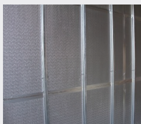
Figure 6: Foil faced PIR insulation board covered with furring prior to installation of plasterboard (photo courtesy of Reflex Insulation Pty Ltd).
